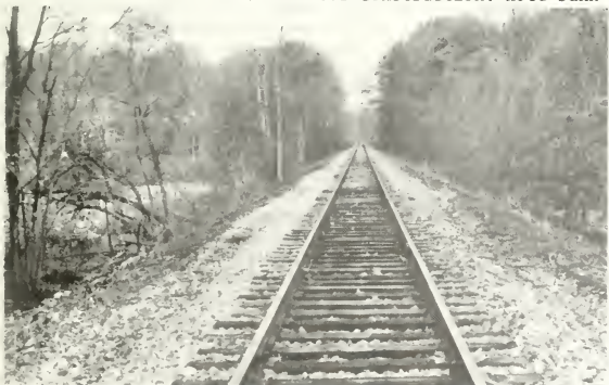
Figure 11. Railroads were built across the ponds and swamps, and their embankments modified drainage: originally, there were open trestles a mile or more in length across the lowest sites, but now those are mostly filled; the above view is the Burlington Northern where it crosses Heron Pond
