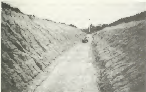
Figure 10. Looking south along a ditch cut across a low ridge to drain farmland straight south into the Cache, one mile west of Cypress Creek Ditch; photo was taken one year after construction: note bank erosion
